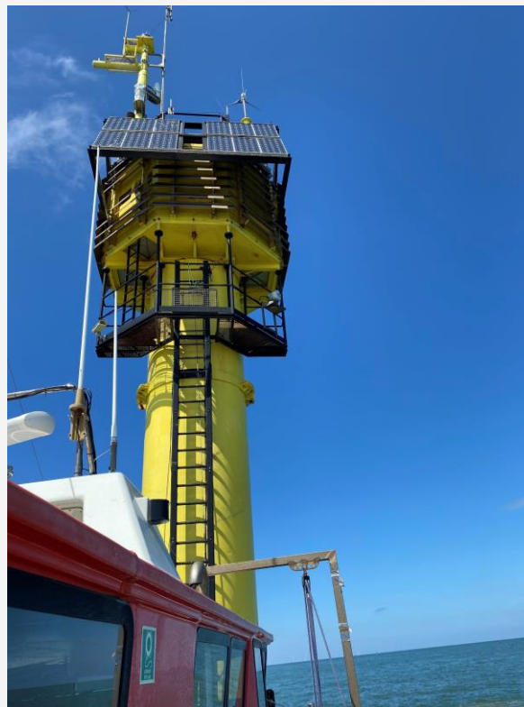
Installation of GNSS antennas on North Sea
