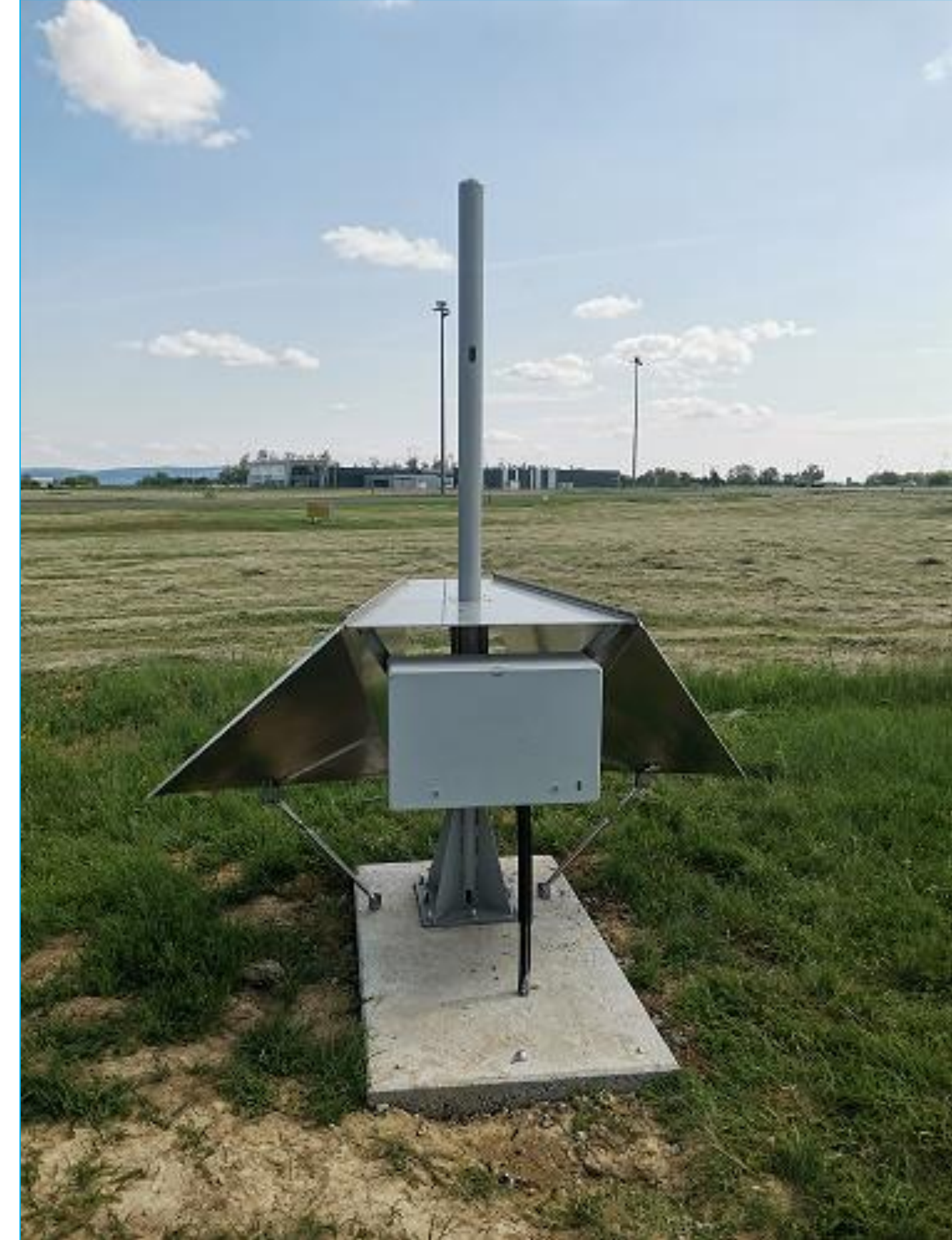
MPOG – steel mast and radar corner reflectors (Airport, Pécs-Pogány)
