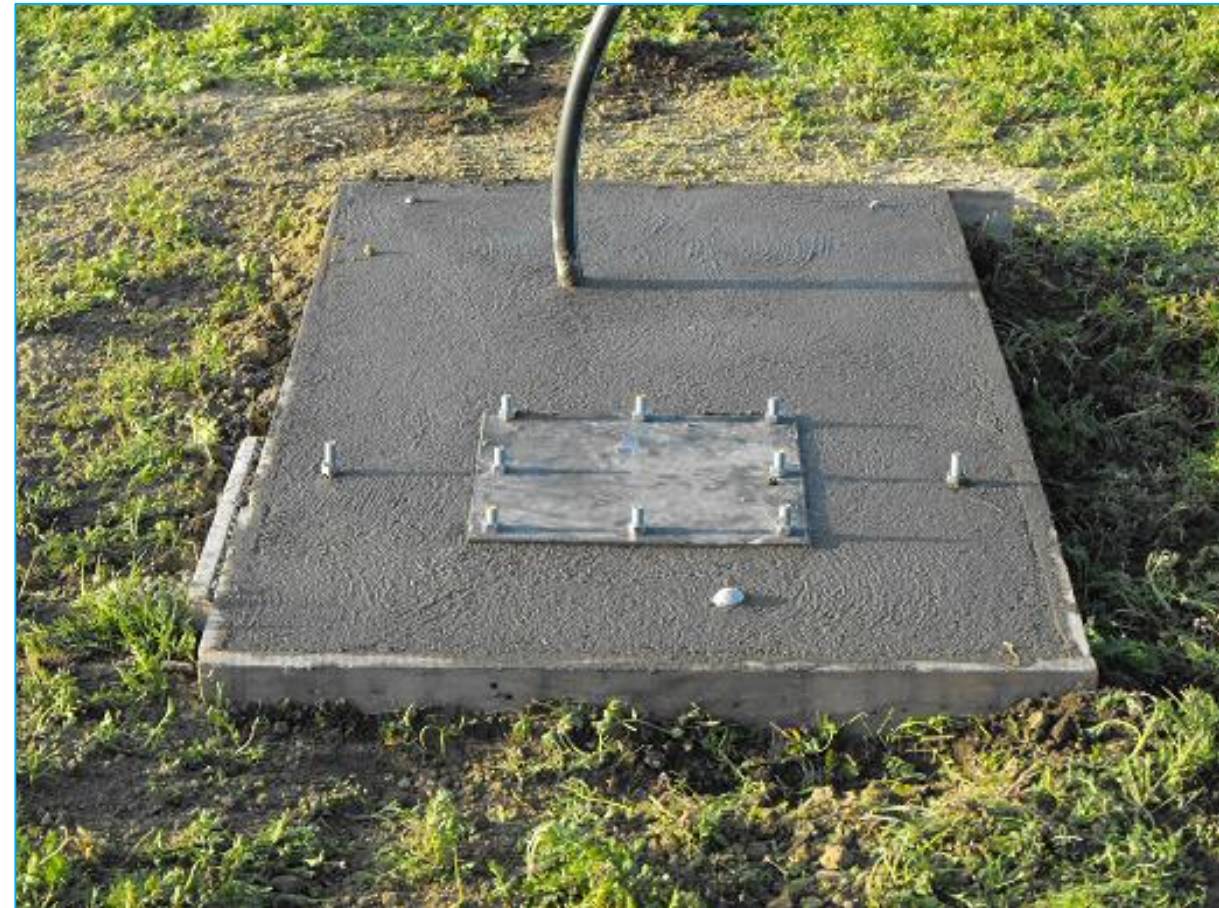
Stable foundation → concrete block: depth: 1.4 m; length: 1.4 m; width: 0.8 m
