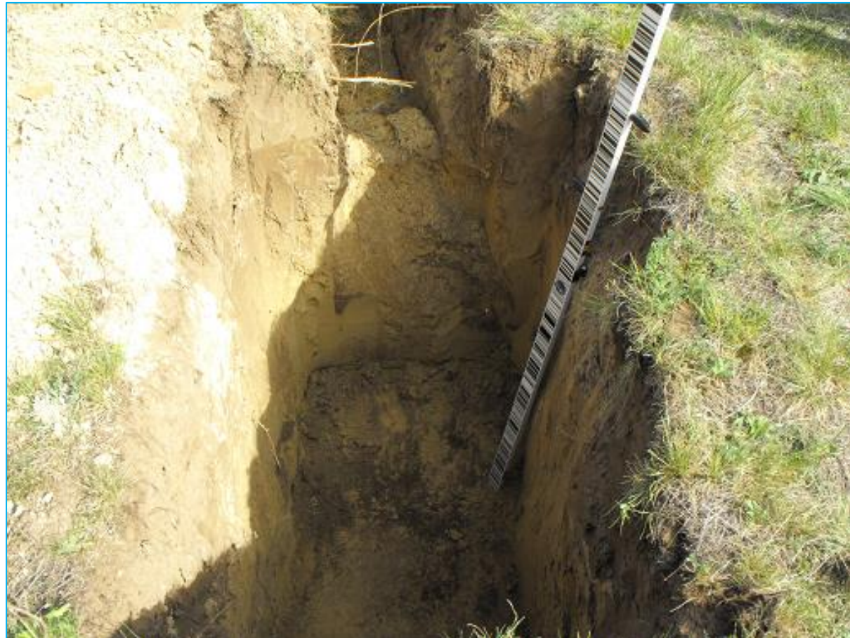
Stable foundation → concrete block: depth: 1.4 m; length: 1.4 m; width: 0.8 m
